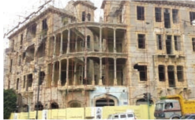
Above: The 'Beit Beirut' building which was used as a control post and sniper base during the civil war and is now being converted into a museum and a cultural and artistic meeting place.
